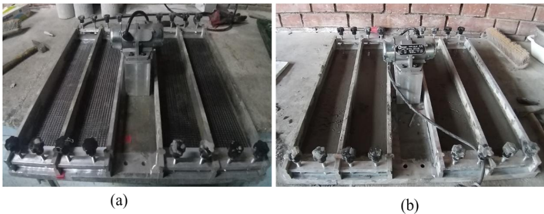
Figure 3-13 C-TRCC formwork: (a) textile placement in the forms (b) placement of cementitious mortar
